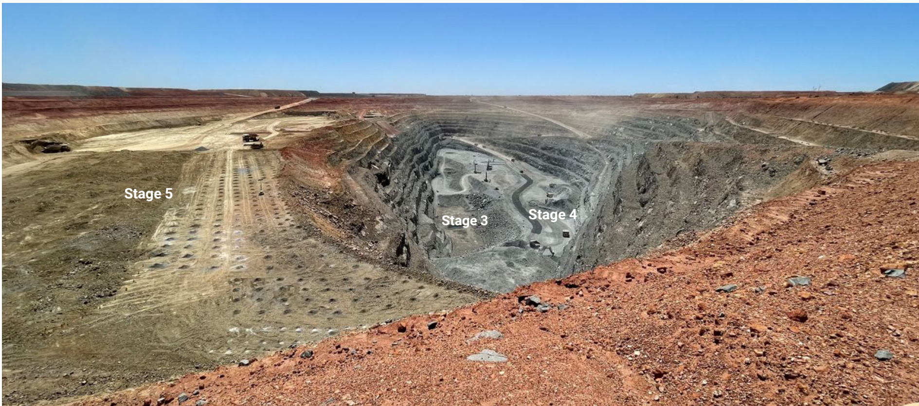
View looking north into Open Pit showing Stage 5 cut-back and Stage 3 & 4 pits – 24 October 2024
