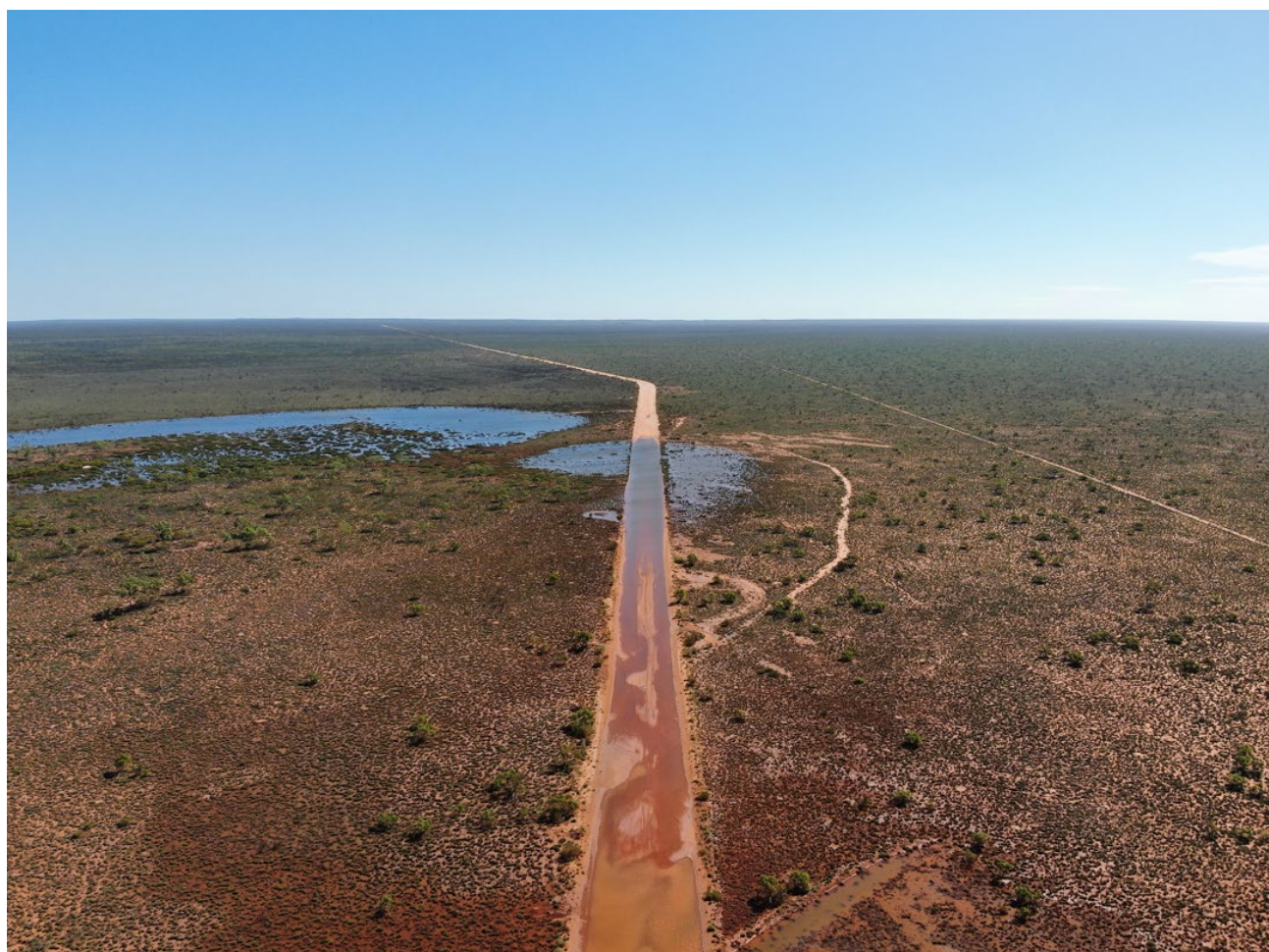
Figure 1: Great Central Road Flooding 20 March 2024
