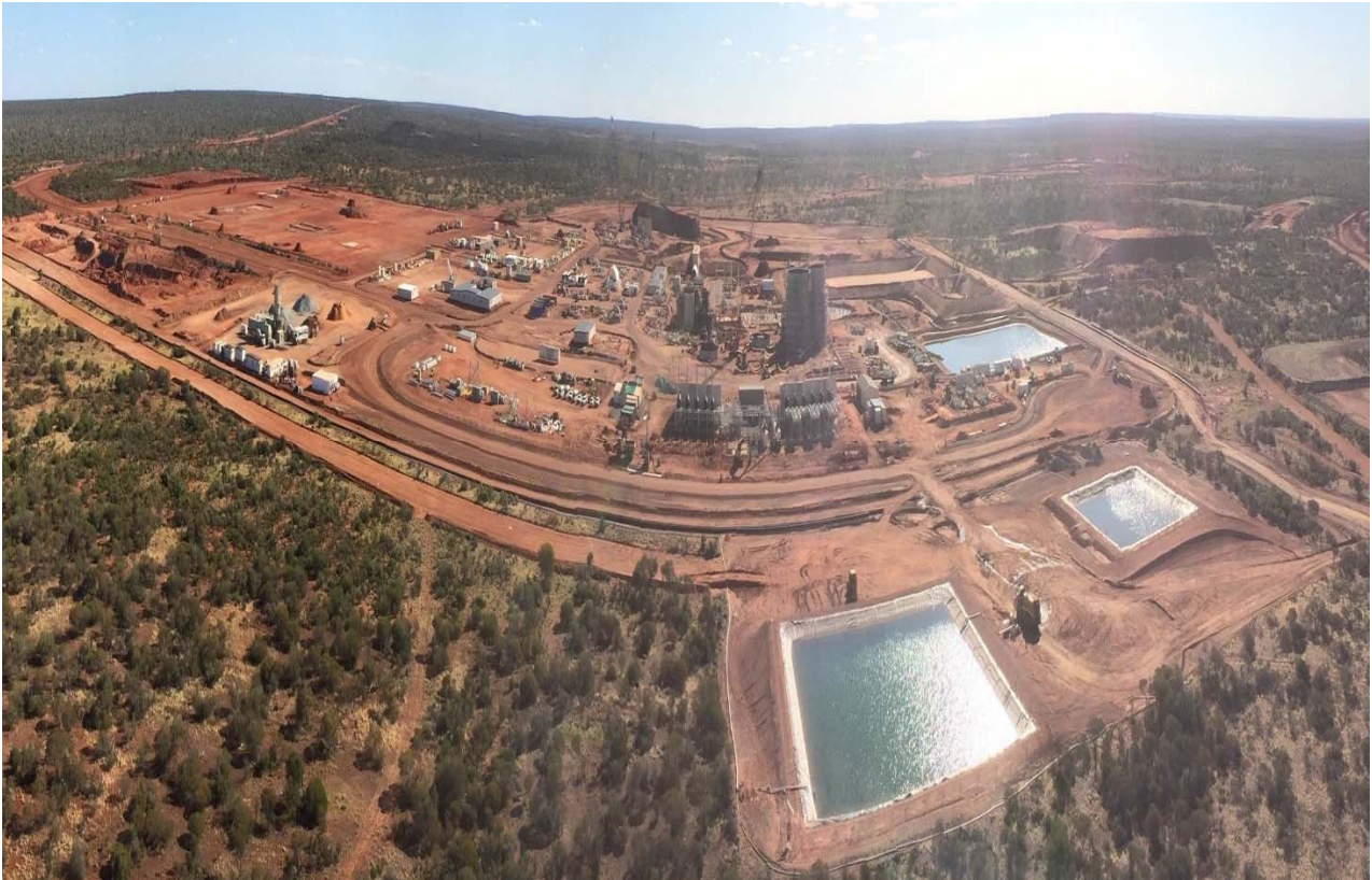
Milling and CIL Tanks
