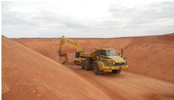
Primary Crusher – Excavation of Raft Foundation
