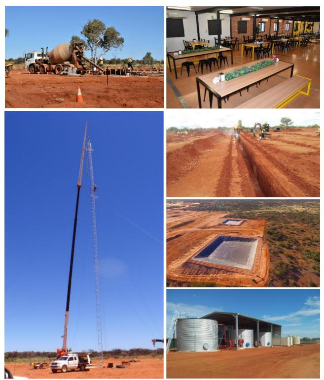
Clockwise from top left - Gruyere Village Stage 1 pad construction; Completed Gruyere Village dining room; Trenching for underground service Gruyere Village Stage 1; Process Plant and Turkeys Nest aeriel view; Gruyere fire water services; Erection of the Gruyere communications tower.
