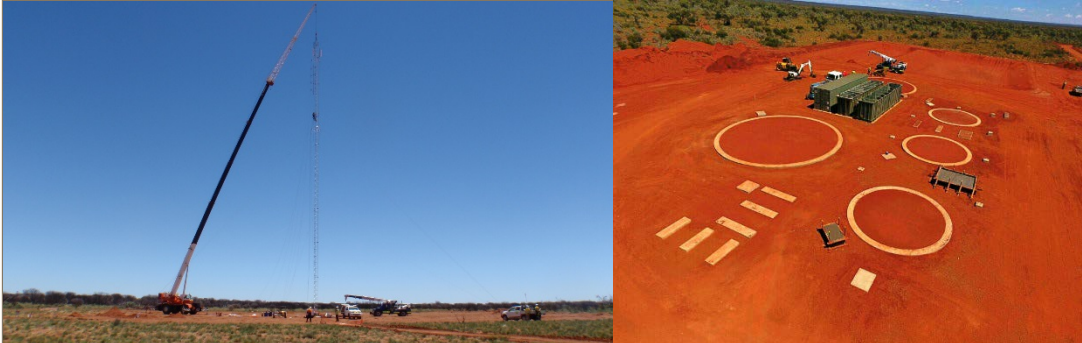
Construction of infrastructure underway
