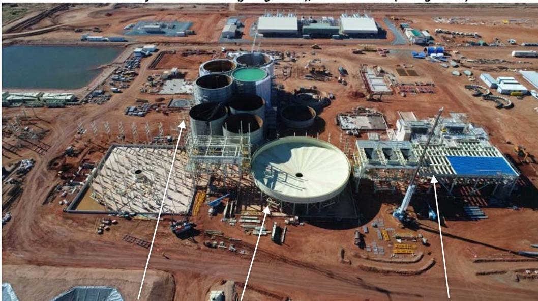
***Aerial view of CIL tanks, pre-leach thickener and base structure for the SAG and Ball Mills***
