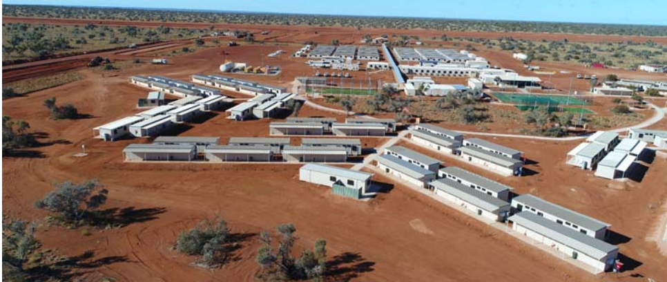
Completed Gruyere Village
