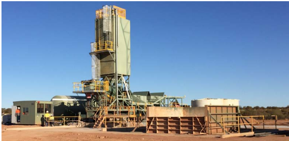
Newly installed Concrete Batch Plant
