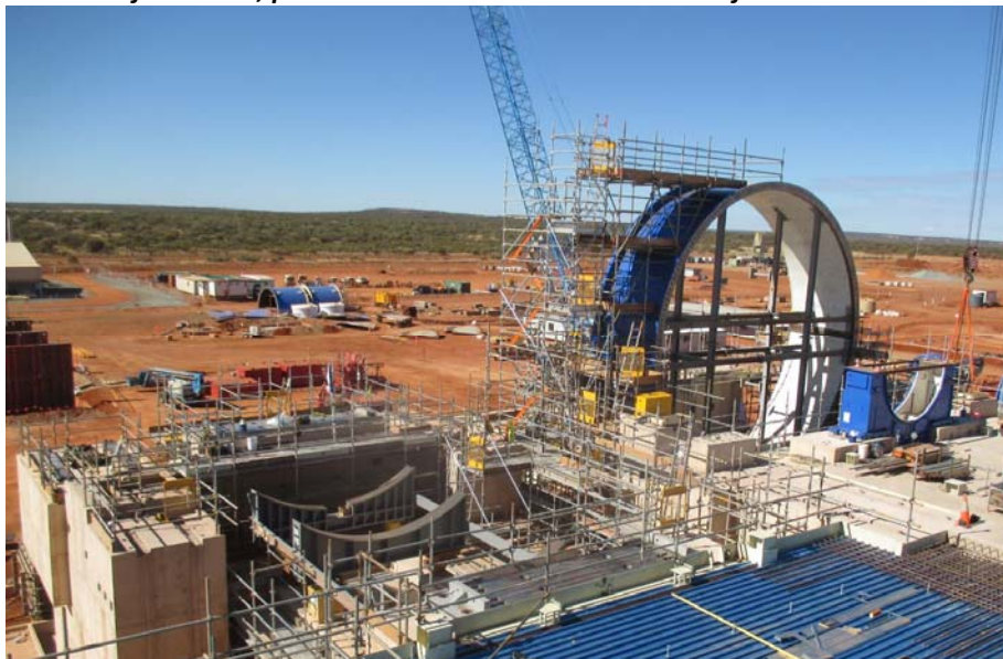
Installation of SAG and Ball Mills
