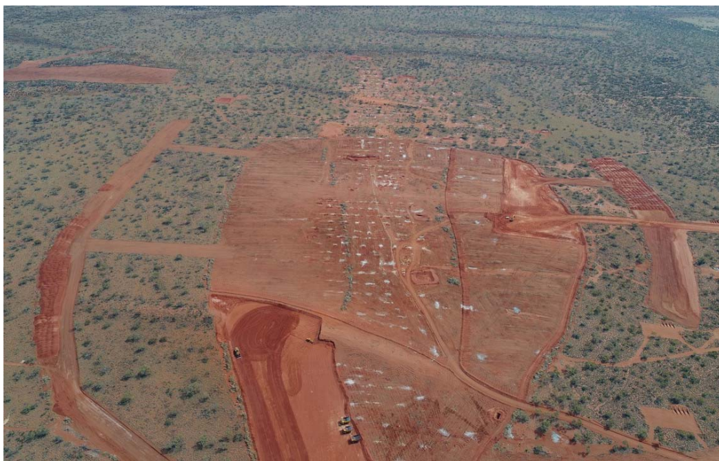
Gruyere Stage 1 pit clearing
