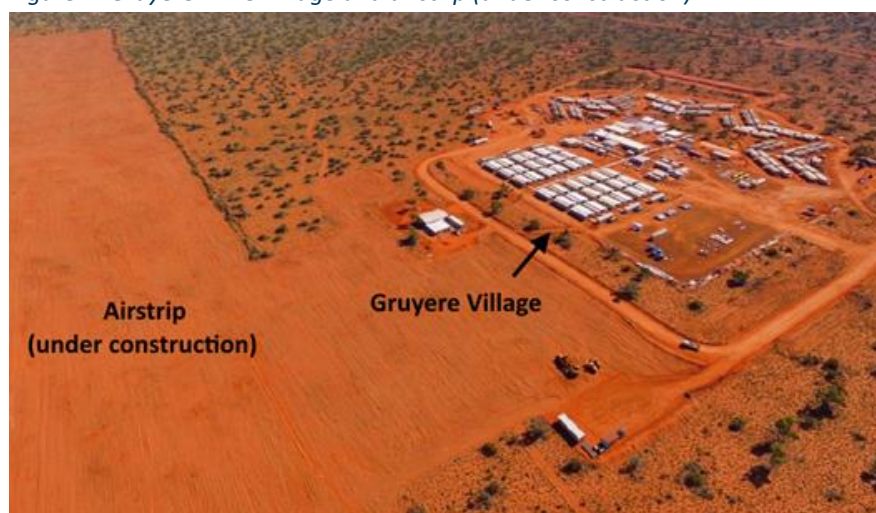
Figure 2: Gruyere Mine Village and airstrip (under construction)
