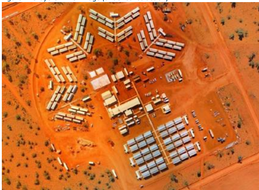
Figure 1: Gruyere Mine Village (under construction)
